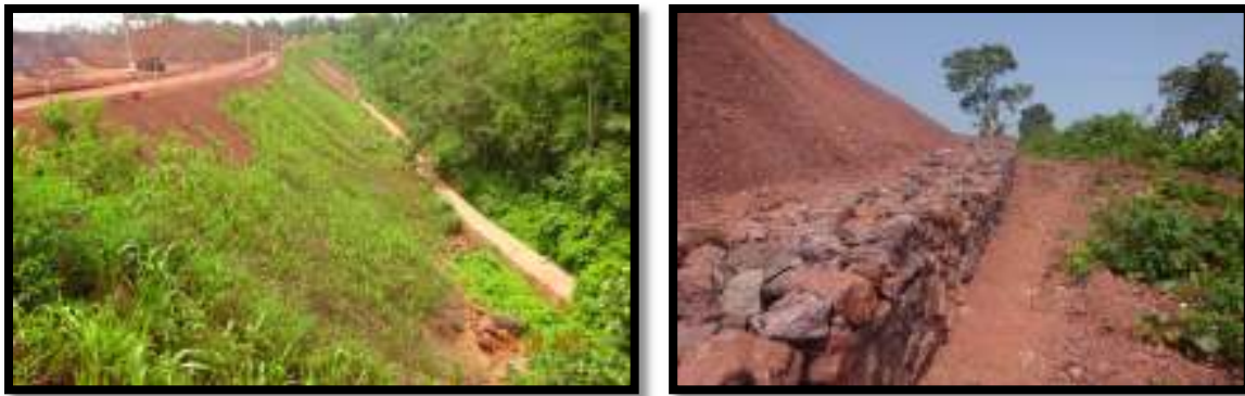
Retaining wall provided at the toe end of the dump
