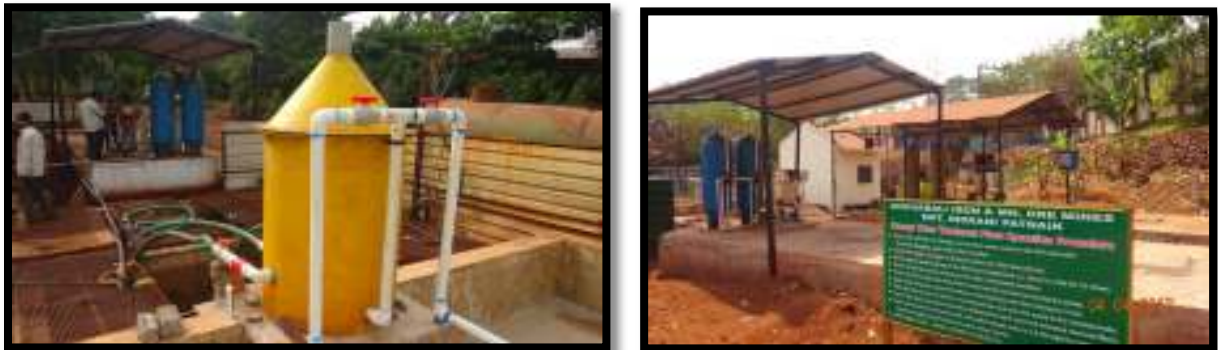
PHOTOS SHOWING STP TECHNICAL STRUCTURE & EXISTING PLANT
